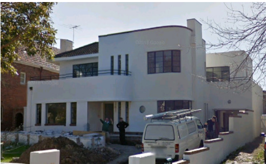
HO189 15 Walbundry Avenue, Balwyn North, Individually significant in Riverside Estate and Environs (Source: Google Maps)
