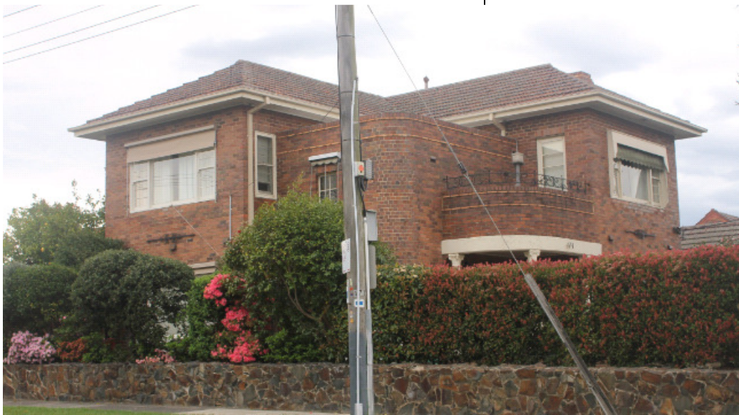
Figure 1. View of 171 Doncaster Road, Balwyn North. (Source: Context, October 2017)
