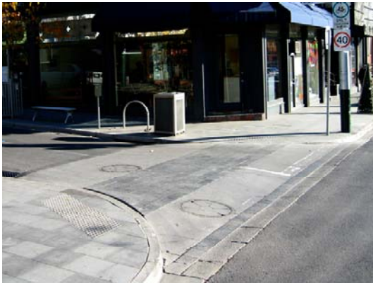
Figure 7. A raised footpath – giving a CTP, in Toorak Road, South Yarra
