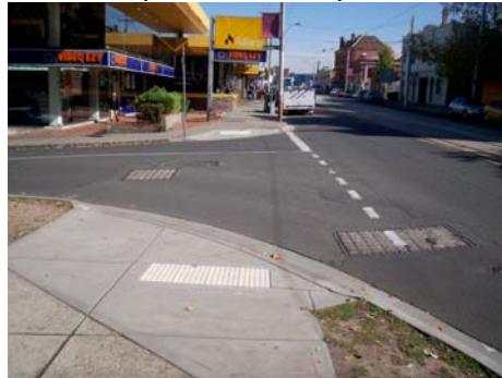
Figure 1. The Pram ramps and tactile plates at Gellibrand Street.
