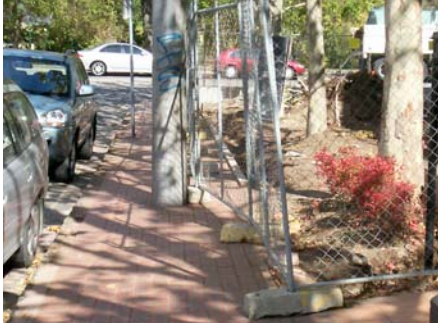
Figure 11 The footpath with a pole in the middle – Derrick Street
