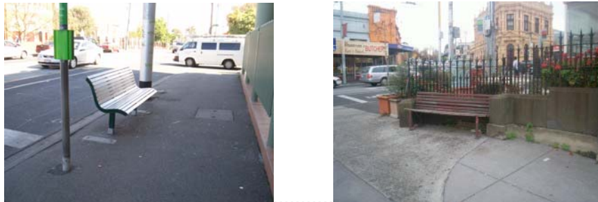
Figure 3. A variety of seat designs - some of which need repair.
