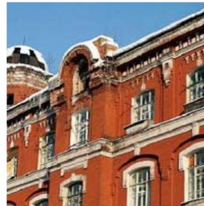
6. Heritage emphasising red brick
