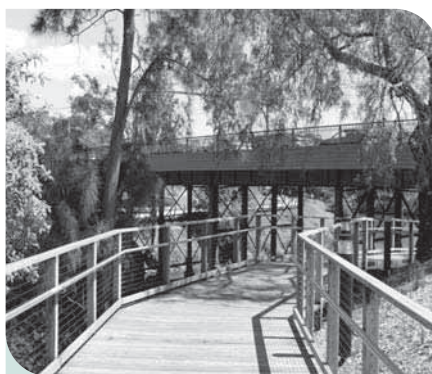
The new pedestrian and cyclist boardwalk at Leonda by the Yarra.
