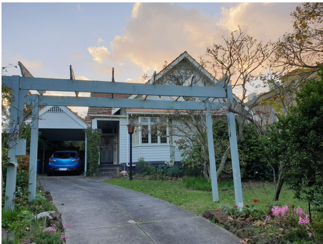
Figure 10. Principal elevation of 5 Creswick Street, Deepdene. Note the canted bay window with leadlight casement sash window, window hood, brick and roughcast rendered porch pier and Federation-style front door surround. (Source: GML 2021)
