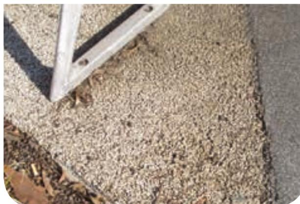
Permeable surfaces enable water to flow into the soil and eventually the groundwater
