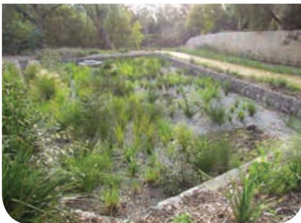
**Image 1** Hambledon Street raingarden treating stormwater before it enters the Yarra River
